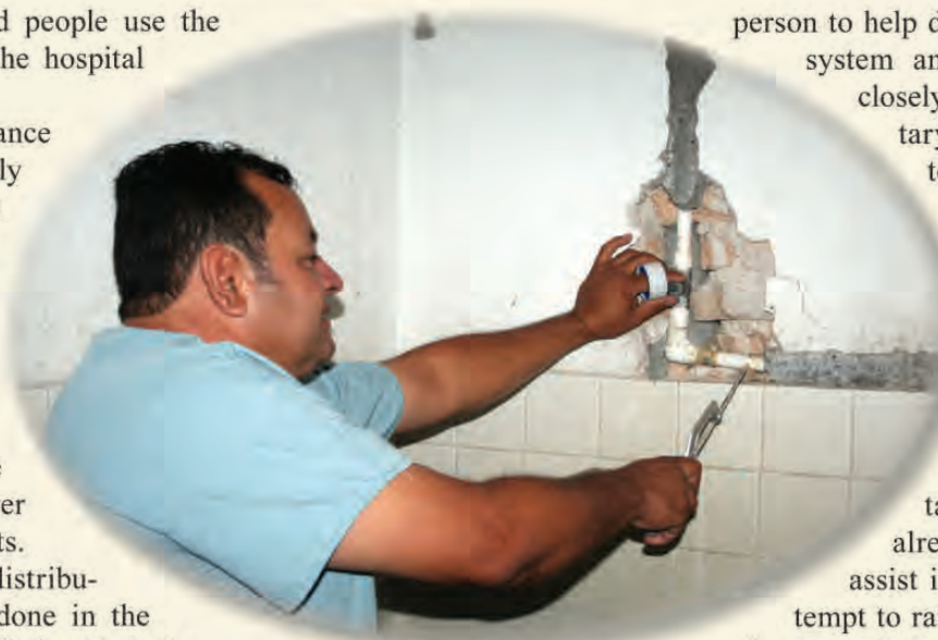
The water distribution system within the hospital is in desperate need of an update
