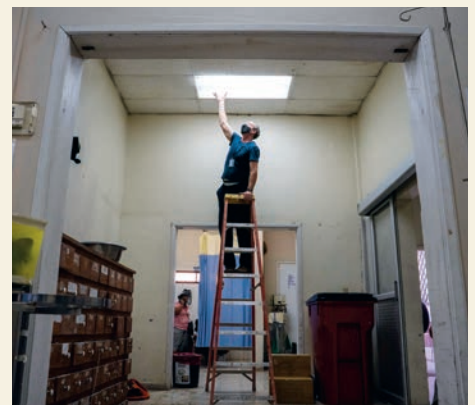
Patrick, US volunteer, replacing lights in the emergency room.
